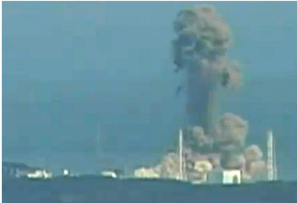
Figure 3. Possible steam explosion in the Unit 3 at the Fukushima accident.
