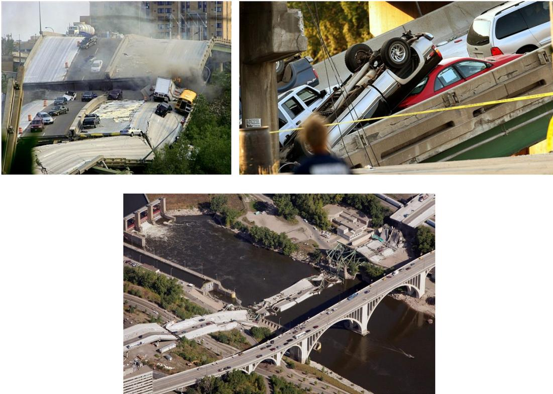
Figure 1. Collapsed 40 years old Minneapolis I-35W highway on the Mississippi River Bridge, August 1<sup>st</sup>, 2007, killed 13 commuters and injured 145 motorists. A new bridge was built on the same spot at a cost of \$250 million and reopened on September 18, 2008. The Federal Highway Administration (FHA) suggests that one in four of the more than 600,000 bridges in the USA are either "inadequate" or outdated.
